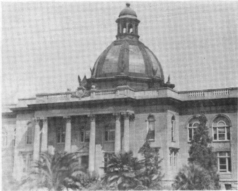
Courthouse #4, the building in use today, circa 1920
