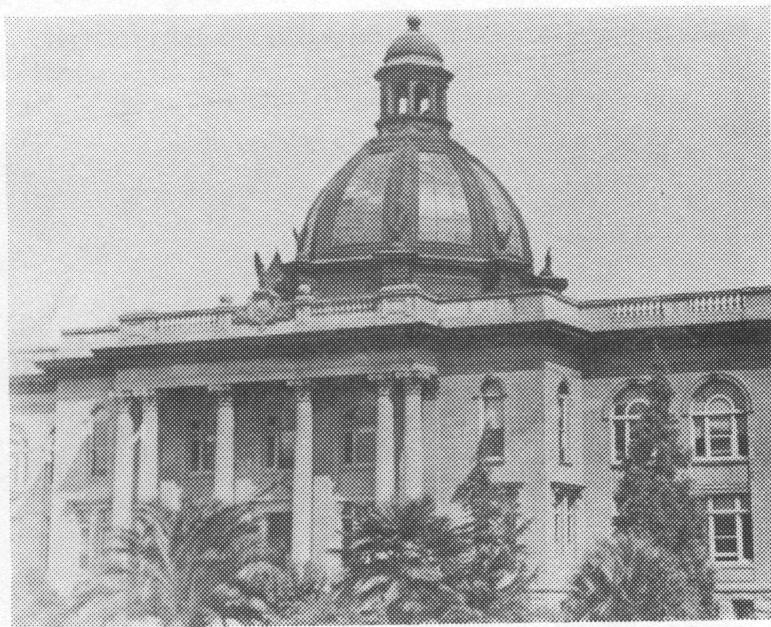
Courthouse #4, the building in use today, circa 1920
